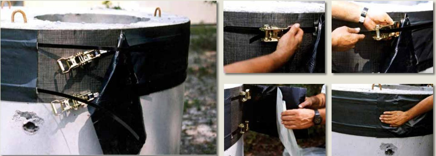
**Step 1:** Brush or sweep portion of joint to insure foreign materials do not interfere with the direct contact between the joint to be sealed and the mastic sealer of the CRETEX WRAP.
