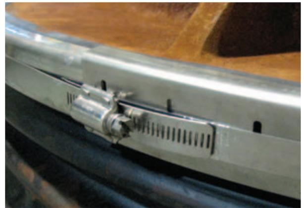
Our unique "C"-shape band mechanically locks the seal on the manhole casting for lasting performance. Our high-performance seal requires no primers torches or special tools to create a watertight barrier.
